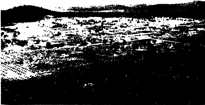
FIG. 30. STANTHORPE, SOUTH QUEENSLAND
